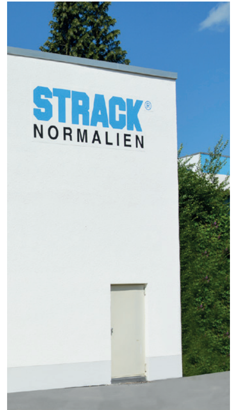
Since June STRACK NORMA tests pressure equipment inhouse in the new test hall.
